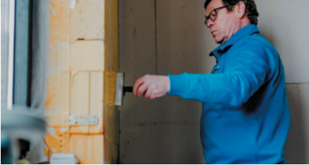
Step 3: Saw to width
