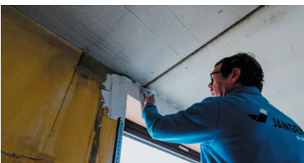
Step 7: Plaster adjacent walls
