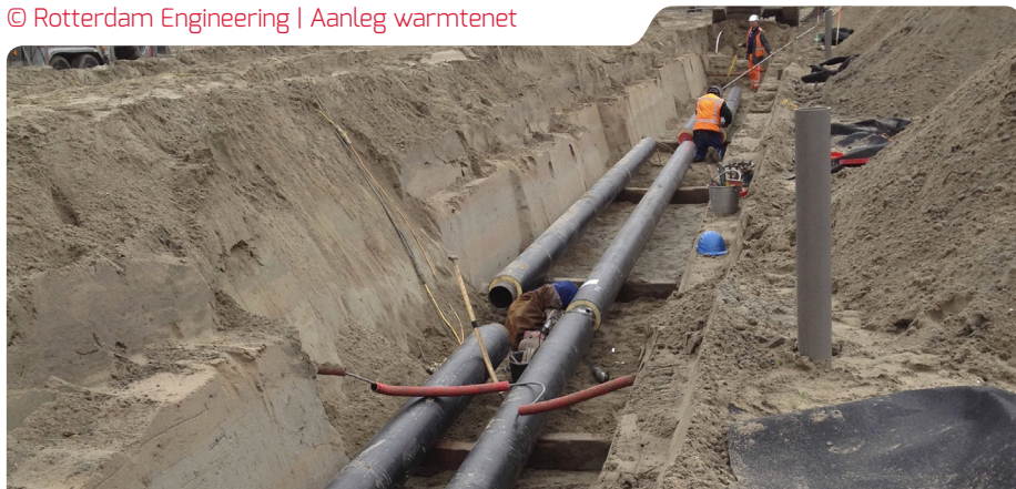
© Rotterdam Engineering | Aanleg warmtenet
